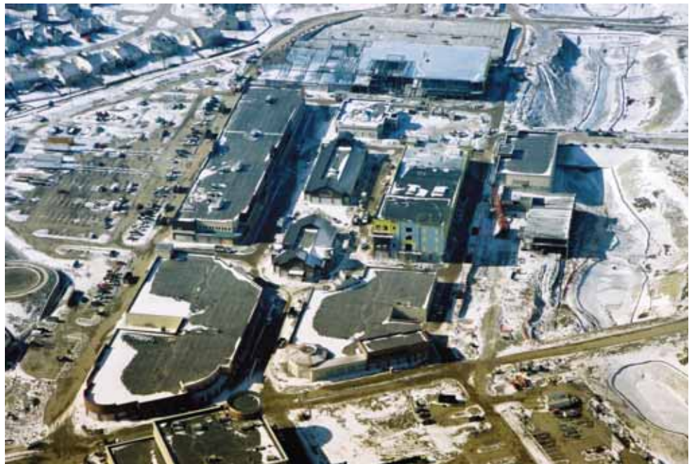
Zona Rosa during construction.
