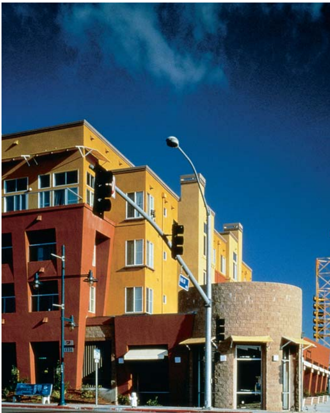
Multifamily housing is better designed than in the past. Bridgecourt in Emeryville, California, brings high style to a mixed-income community.
